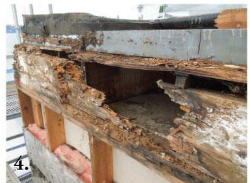
Finding wood rot in a home near a new leak does not necessarily mean that a new water event / claim is long-term. However, if there is extensive wood rot, as shown above, it may be difficult to counter the denial. Pick your battles.
