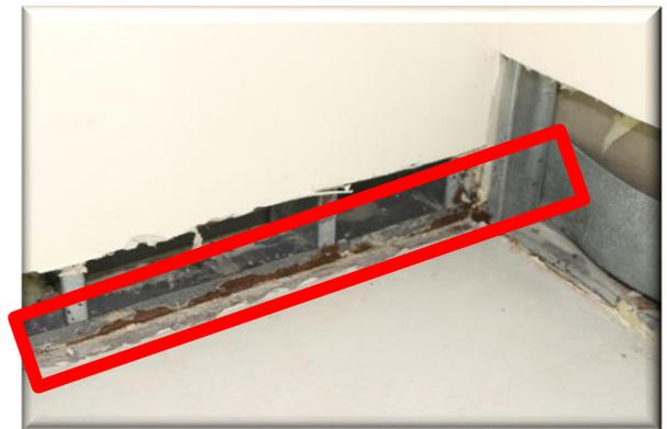
For example, the picture on the right shows heavy rust on a galvanized steel bottom track in an area that was not affected by a new water leak. The exact timing of the new leak was known because it came from a burst water line in the unit above. Since the exact timing of the new leak is accurately known, we can conclude there is previous rust not related to the recent water event.
