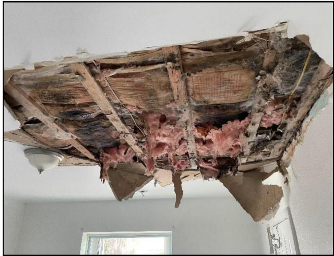
Collapsed drywall ceiling in the bedroom of Apartment 6.
