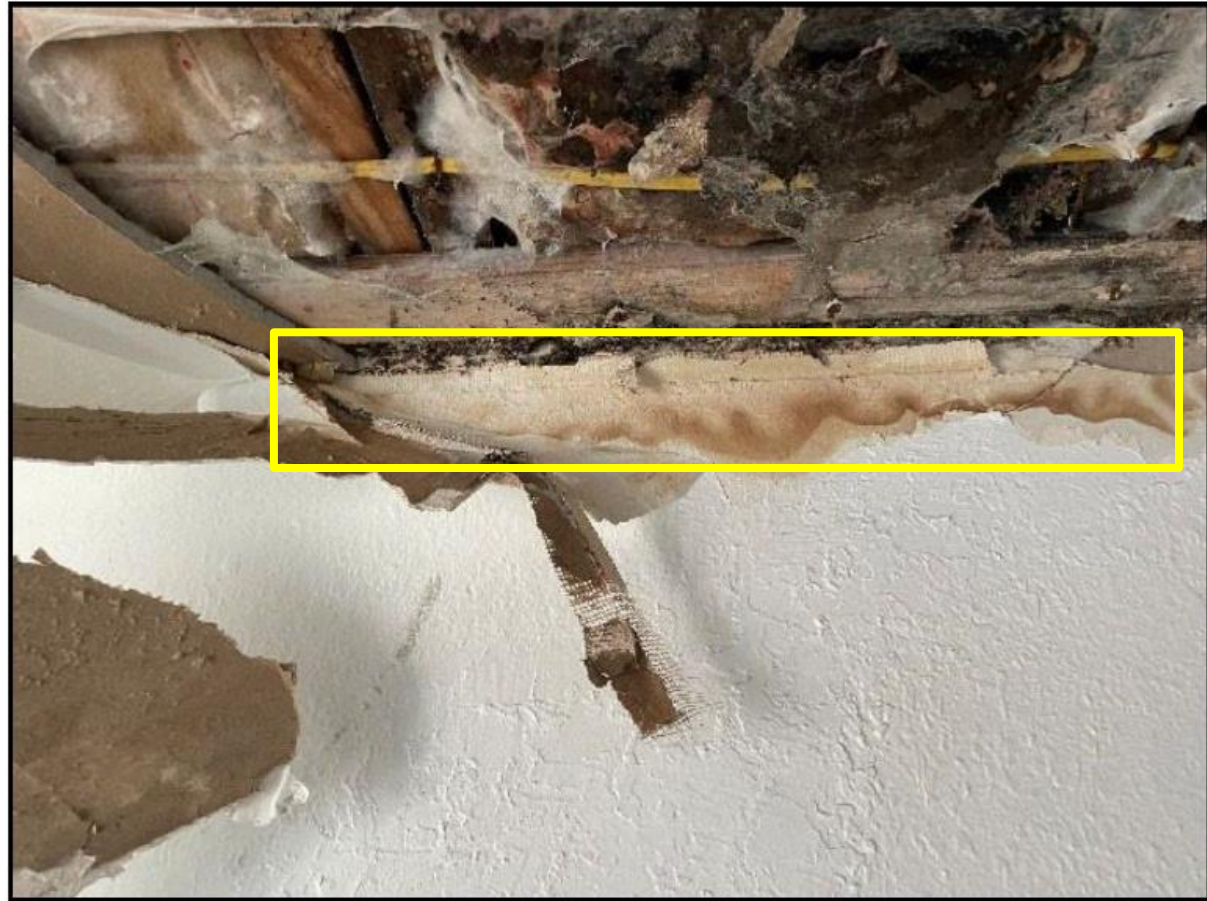
Drywall wall in the bedroom of Apartment 6 with staining.
